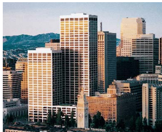
One of the premier office complexes in San Francisco's financial district, One Market contains 1.5 million square feet of commercial space.
