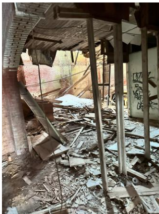
BASEMENT VIEW OF ABOVE FLOOR COLLAPSE
