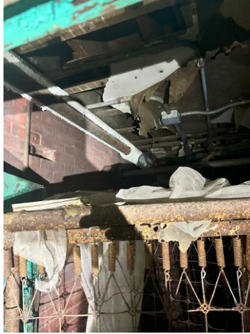
BASEMENT PIPE INSULATION
