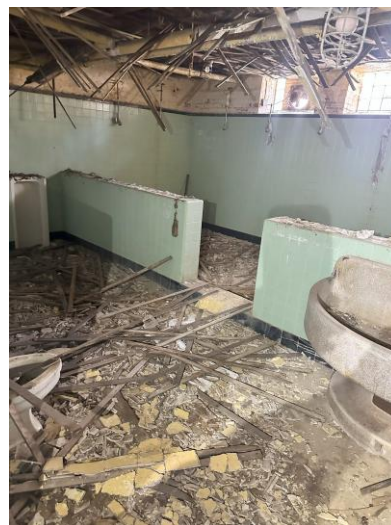
BASEMENT BATHROOM PLASTER PIPE INSULATION THROUGHOUT
