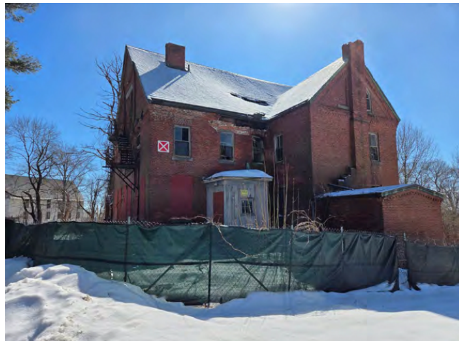
2. WEST ELEVATION, VIEW SOUTHWEST
