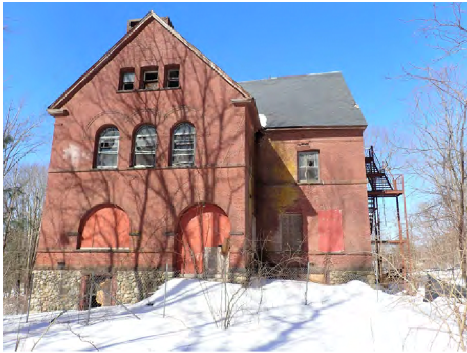
1. SOUTH ELEVATION, VIEW NORTHWEST
