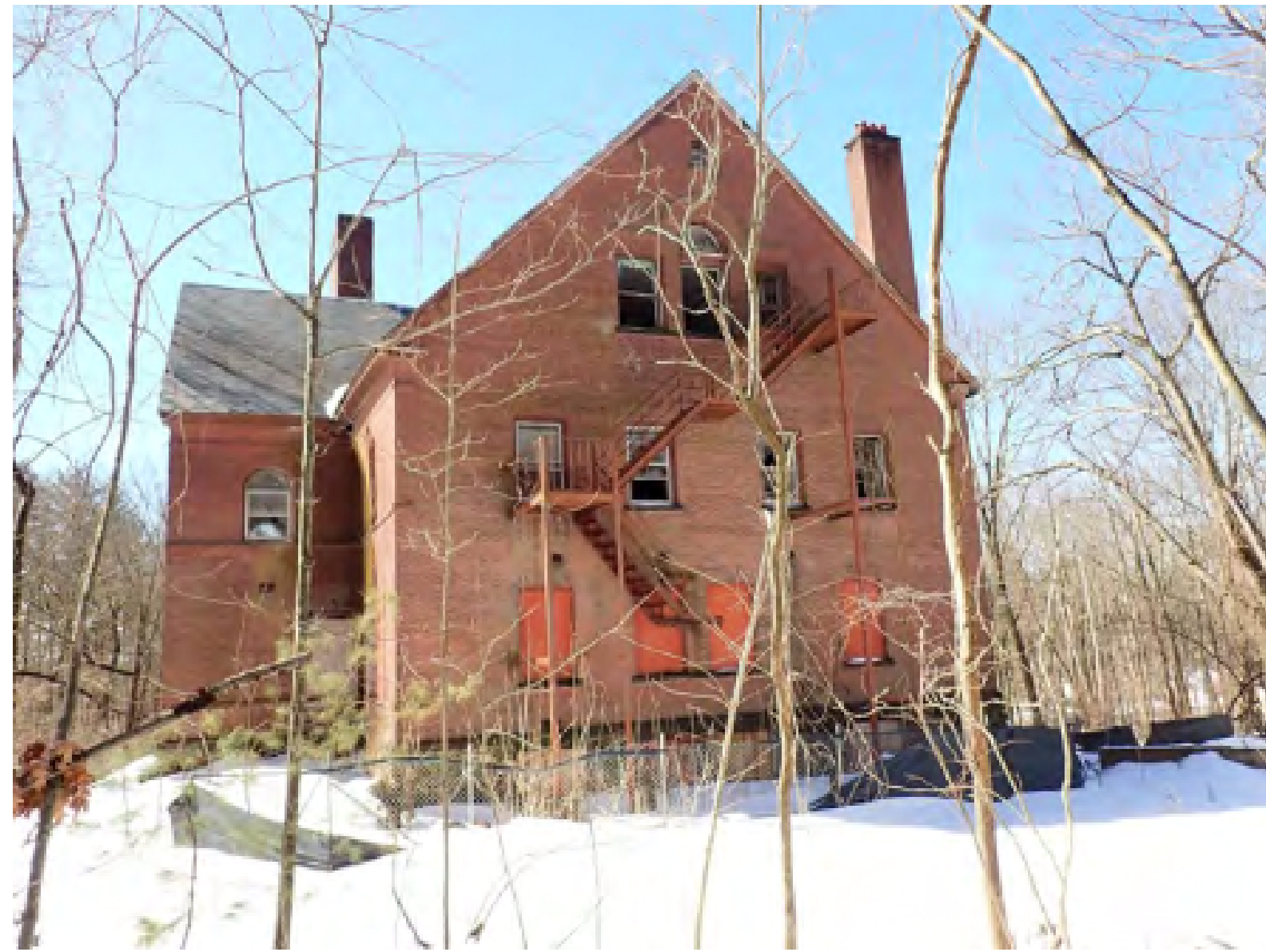
2. EAST ELEVATION, VIEW SOUTHWEST
