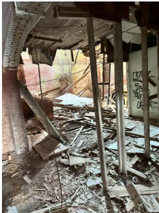
BASEMENT VIEW OF ABOVE FLOOR COLLAPSE
