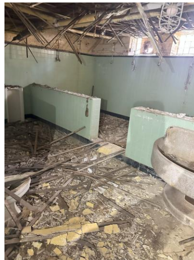
BASEMENT BATHROOM PLASTER PIPE INSULATION THROUGHOUT
