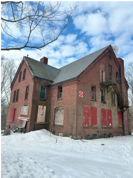
Figure 1 Photographs of the site.
